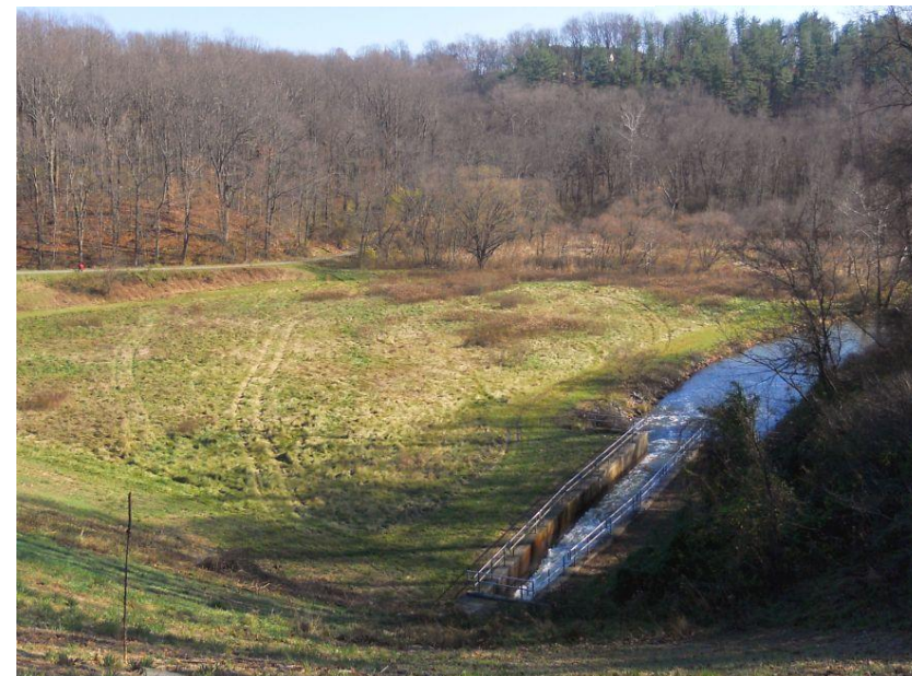
The “floor” of the earthen dam was constructed by boring sixty foot holes in the bedrock and filling them with high pressured cement. As a ecological measure, the Brandywine Valley Association requested the installation of the control tower, which served to monitor the release of water from three different levels. Courtesy of the Brandywine Valley Association
