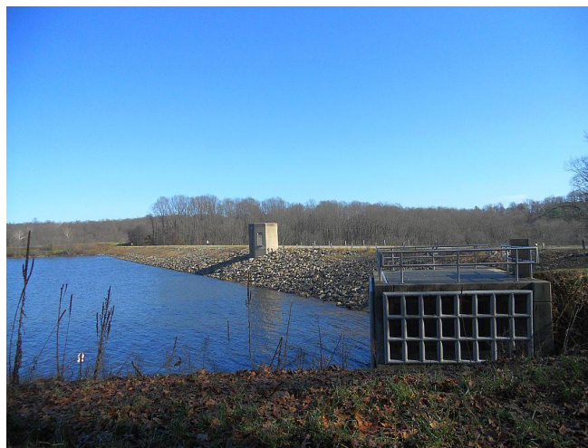
The “floor” of the earthen dam was constructed by boring sixty foot holes in the bedrock and filling them with high pressured cement. As a ecological measure, the Brandywine Valley Association requested the installation of the control tower, which served to monitor the release of water from three different levels. Courtesy of the Brandywine Valley Association
