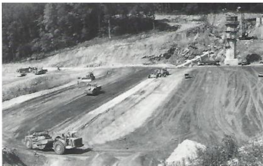
The “floor” of the earthen dam was constructed by boring sixty foot holes in the bedrock and filling them with high pressured cement. As a ecological measure, the Brandywine Valley Association requested the installation of the control tower, which served to monitor the release of water from three different levels. Courtesy of the Brandywine Valley Association
