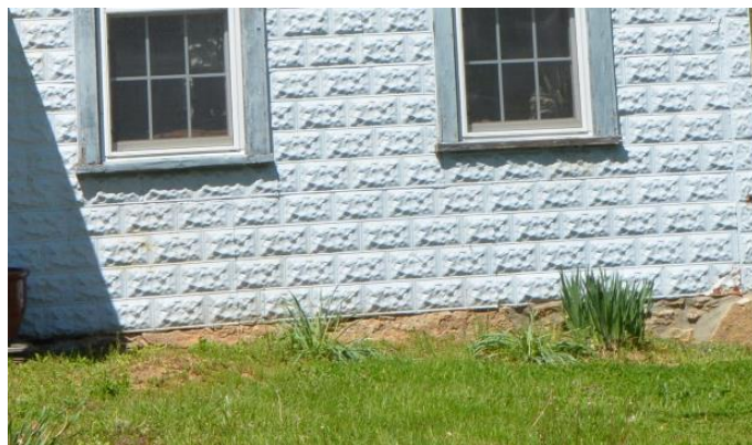
Stone foundation of a wood framed vernacular building (219 Byers Road, Byers Station Historic District). Note: the building is clad in pressed tin.
