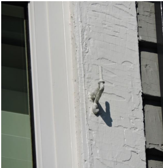
Vestigial historic metal features such as this pintle from a late nineteenth century shutter hinge point to the building's appearance in earlier years.
