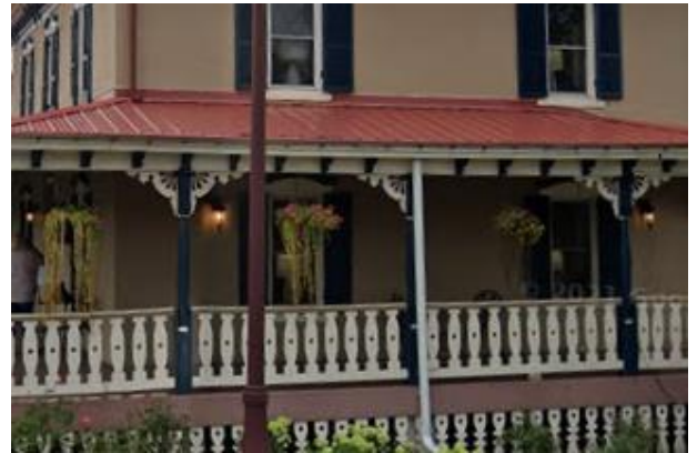
This porch has two-dimensional balusters, which were popular during the 1870s and 1880s. These balusters are character-defining elements of the porch and contribute to the building's original appearance. Also note the skirt enclosing the crawlspace beneath the porch (Sheetz House, 102 Pottstown Pike, Eagle).
