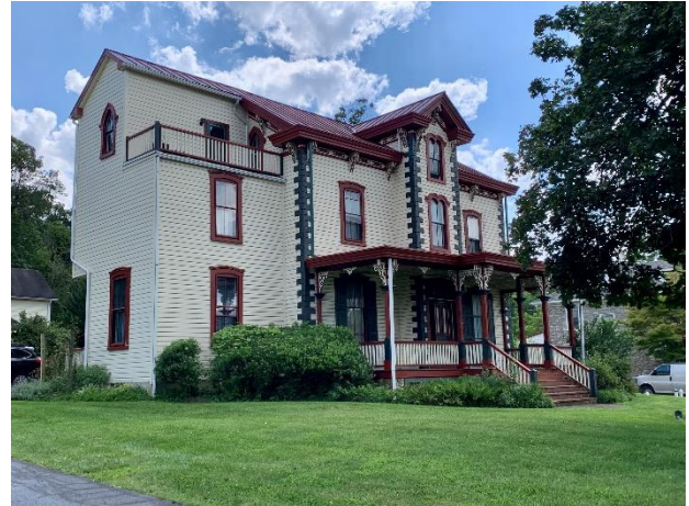
Eastern addition onto the John Todd House in Byers is somewhat compatible with the original design and in fact re-uses the original windows from the openings it covers.
