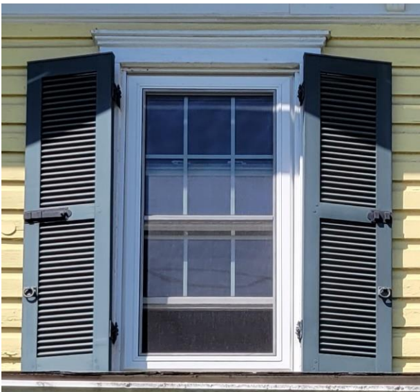
Shutters should match the height and width of the window opening and be operable or at least appear to be operable.
