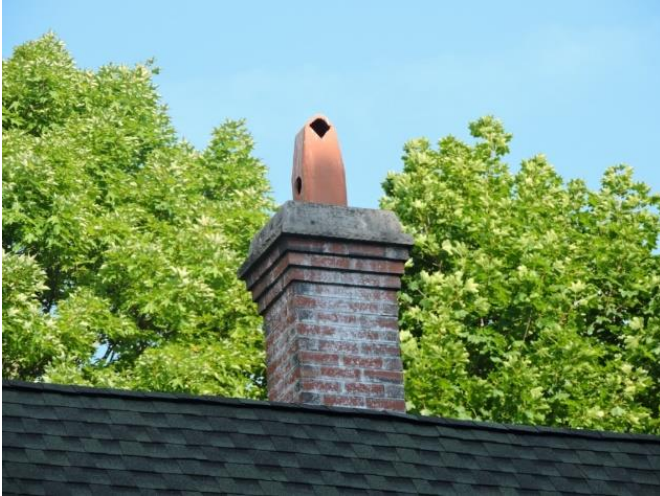
This chimney has a custom stone cap with a terra cotta flue cap.
