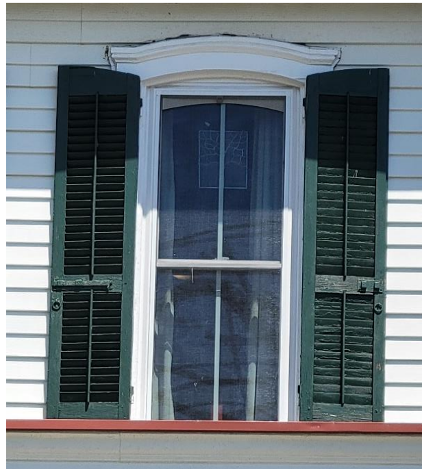
Typical Italianate style, two-over-two sash window with arched head, authentic flanking shutters shaped to fit, and decorative cap trim and surround.
