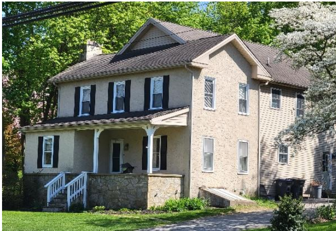
Existing additions located on the rear of the primary historic buildings within the VPA (S.W. Todd House, 236 Byers Road). The addition is in an appropriate location, although its height has altered the historic roofline and is not an appropriate treatment.
