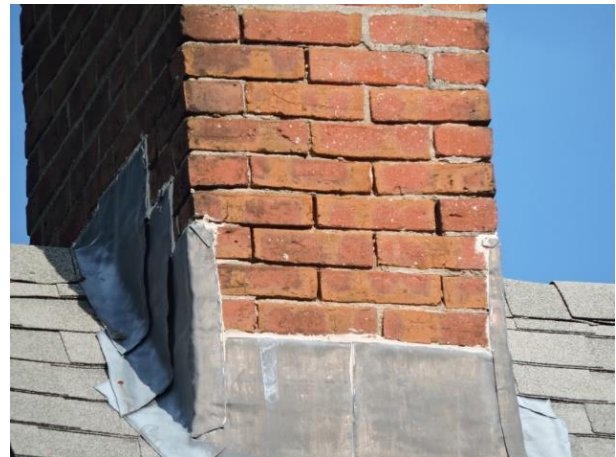
Within the VPA, brick is most often found as the construction material for chimneys, rather than walls. Difficult to access, this brick chimney has open joints which will absorb water.
