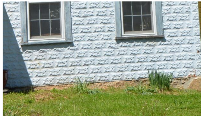
Stone foundation of a wood framed vernacular building (219 Byers Road, Byers Station Historic District). Note: the building is clad in pressed tin.
