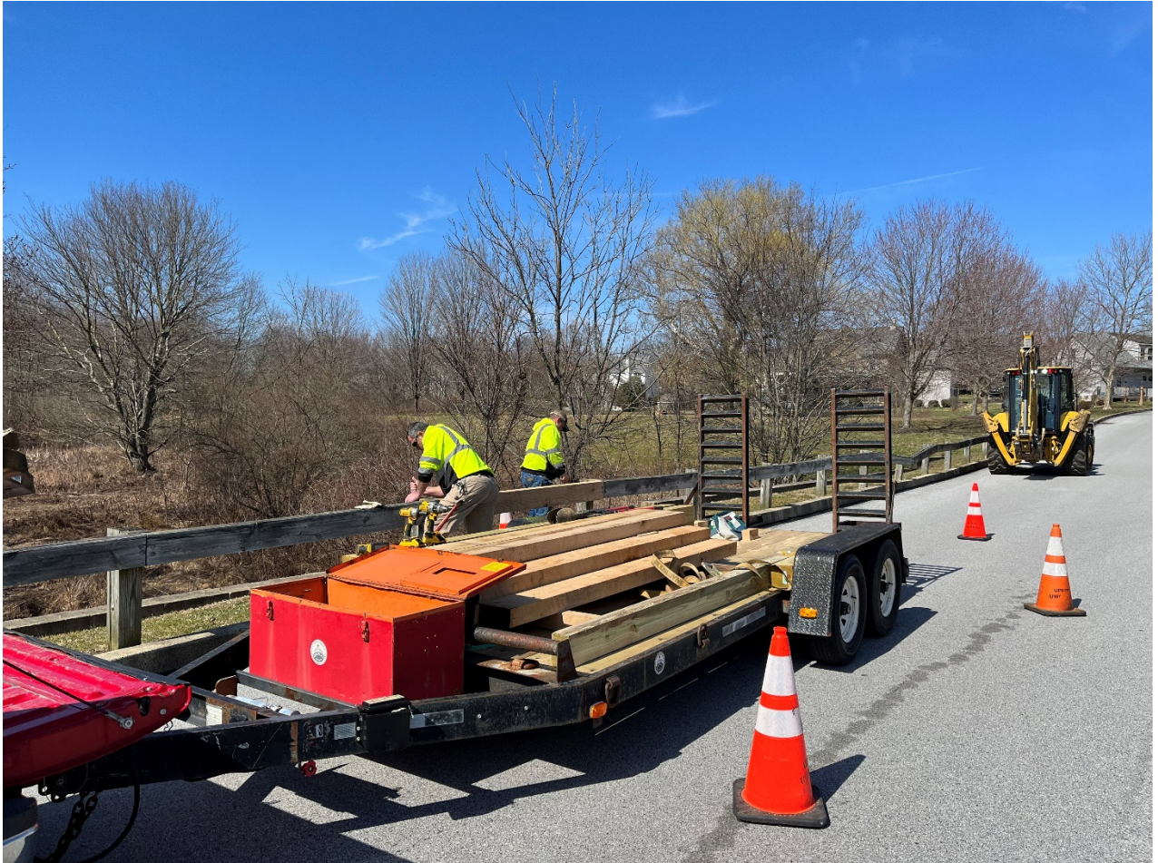
Stanford Road Guardrail Replacement - March 2023
