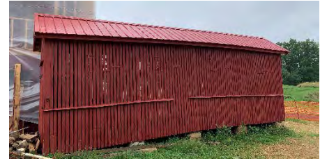
Early in the year, the historic corncrib adjacent to the Barn was restored with fresh coat of paint, replaced slats, and a new roof.
