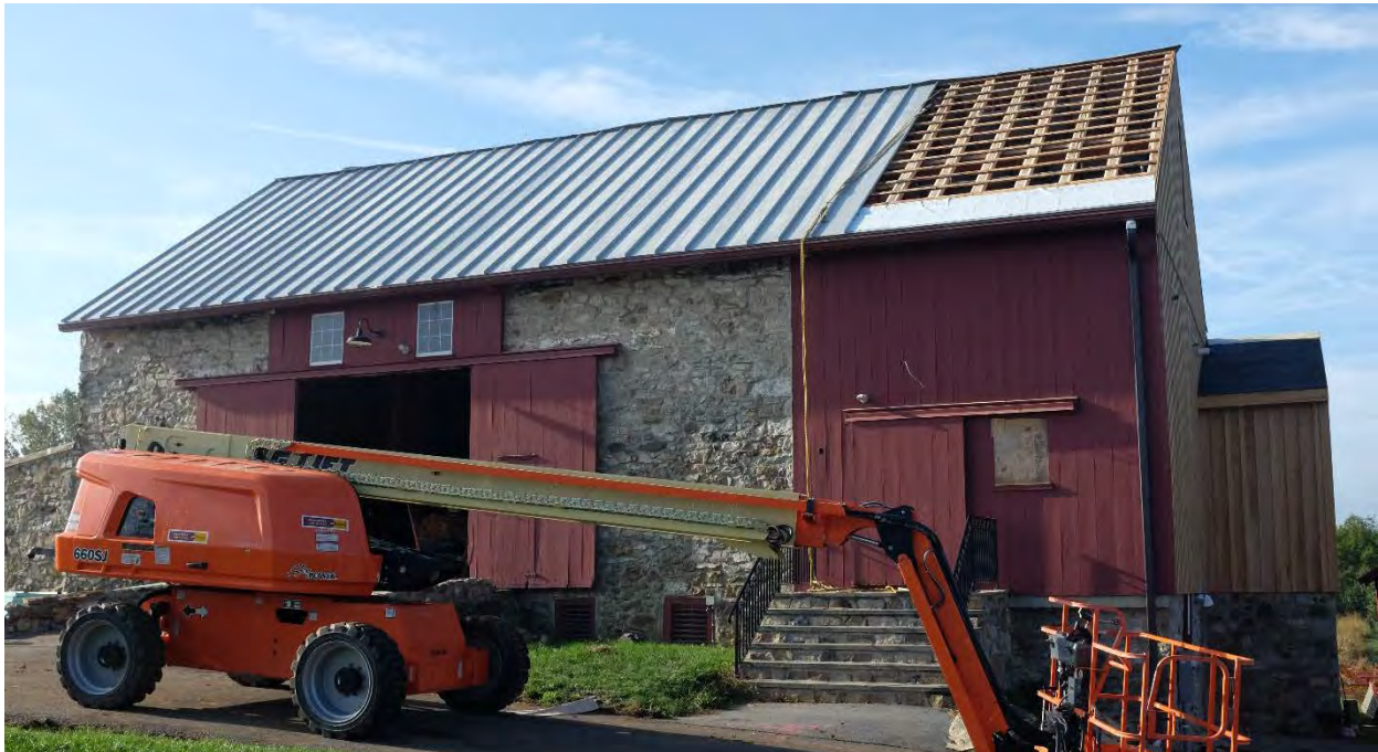
Renovations to the Barn include a new standing seam roof, installed in October.
