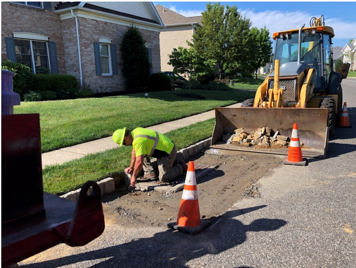
Storm Water Management: Inlet Repair on Prescott Drive
