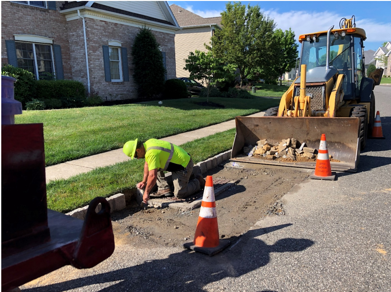
Inlet Repair on Prescott Drive
