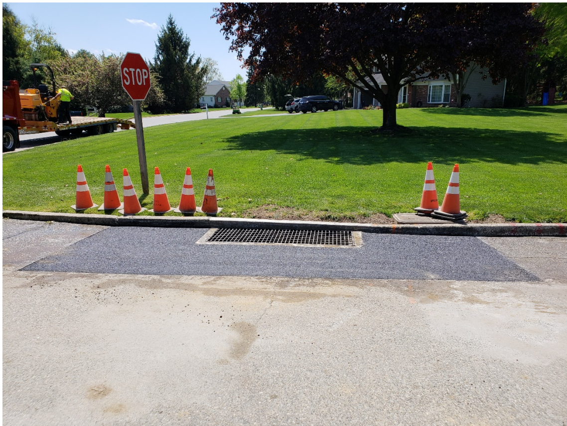
Repairs to a stormwater inlet.
